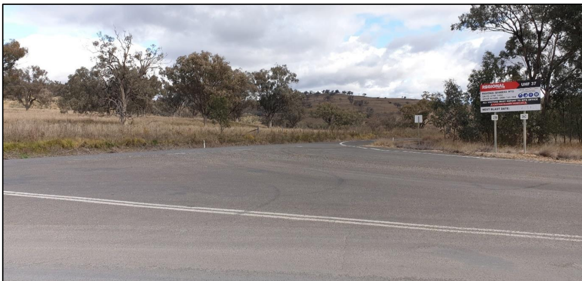
Photograph 1: View south west depicting intersection of Merriwa Road and access road to subject site
